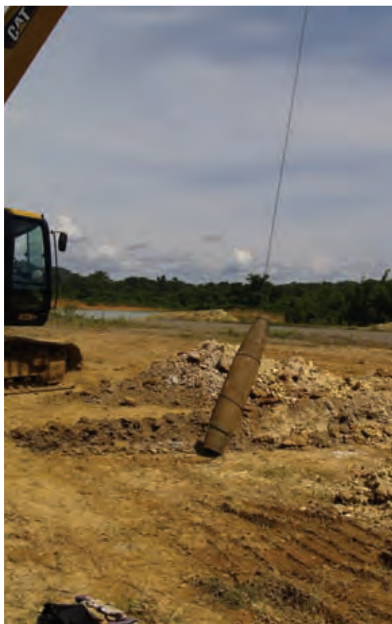
Test Pit Construction
